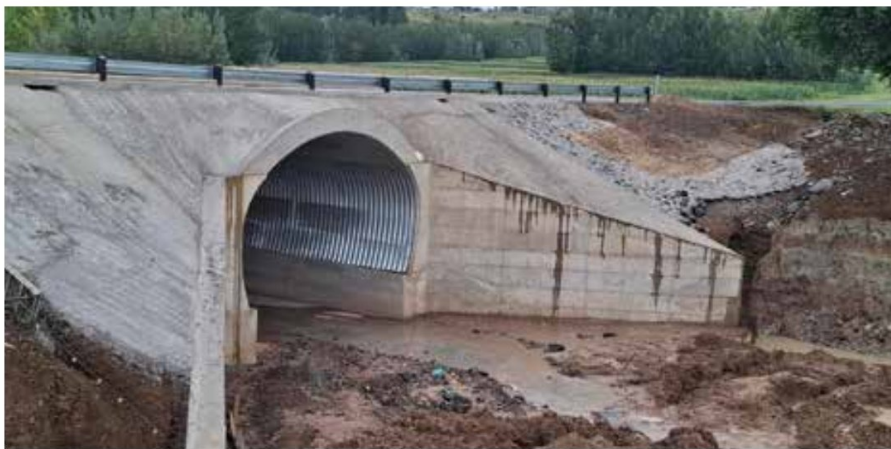
↑ Armco's MP200 structures are used on mining projects as underpass and drainage structures
