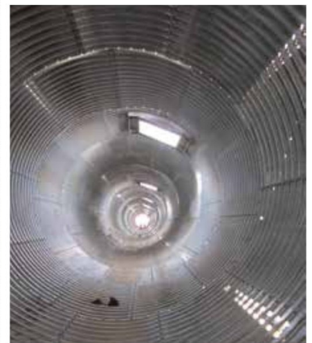
↑ Armco's MP200 structures are used on mining projects as decline, stockpile and reclaim and escape tunnels
